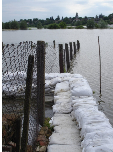
Fig. 2. Flood defence on the Kapos River at Döbrököz, May 2010 (Photo by Lóczy)
